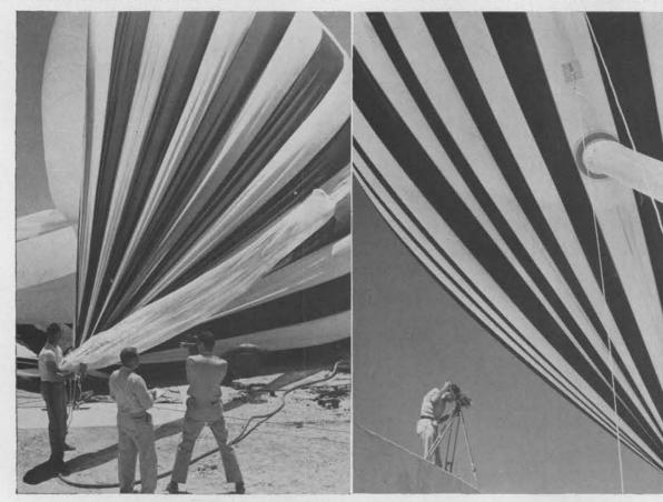
INFLATION is accomplished by inserting a metal probe with thousands of holes into a plastic filler tube attached at the bottom of the big balloon.
